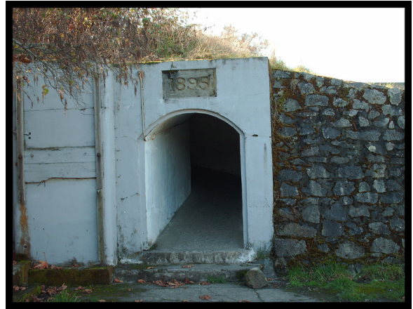
The bottom of the tunnel
